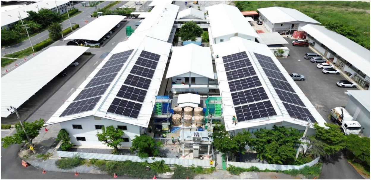
Installation of Solar Panels on the Project Office Building
