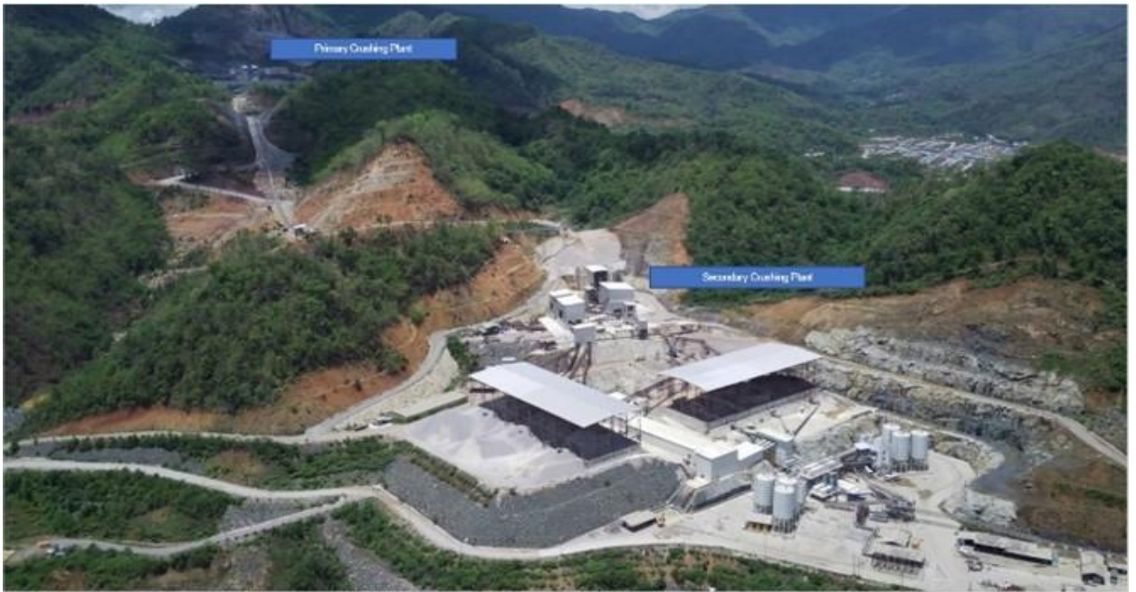
Transportation of Crushed Stone for Concrete Mixing Using Conveyor Belts
